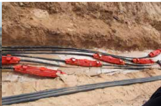
Straight through joints high water table
