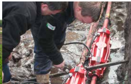
Cross-bonding joints
