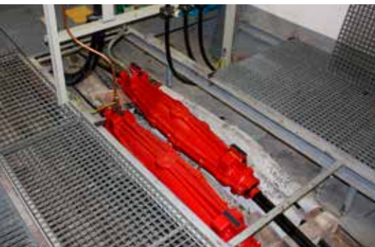
Oil refill joints in switch gear station
