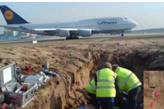
Transition joints Airport
