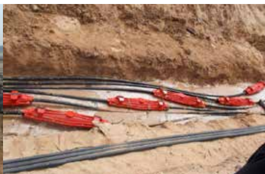
Straight through joints high water table
