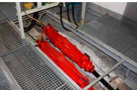
Oil refill joints in switch gear station
