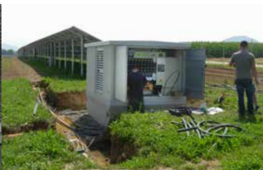
Feed-in splices Solar park
