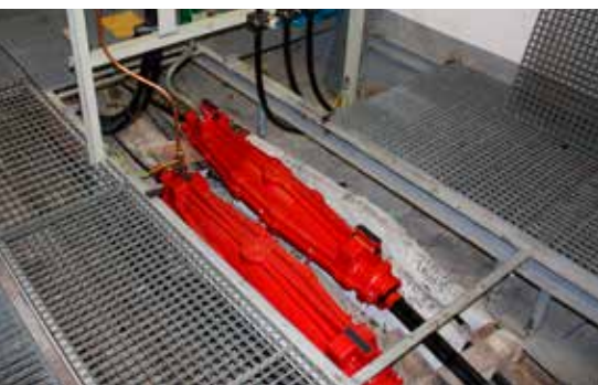
Oil refill splices in switch gear station
