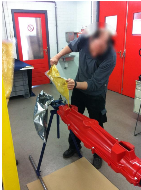
Figure 2. Filling of the cable joint (exp 1)
